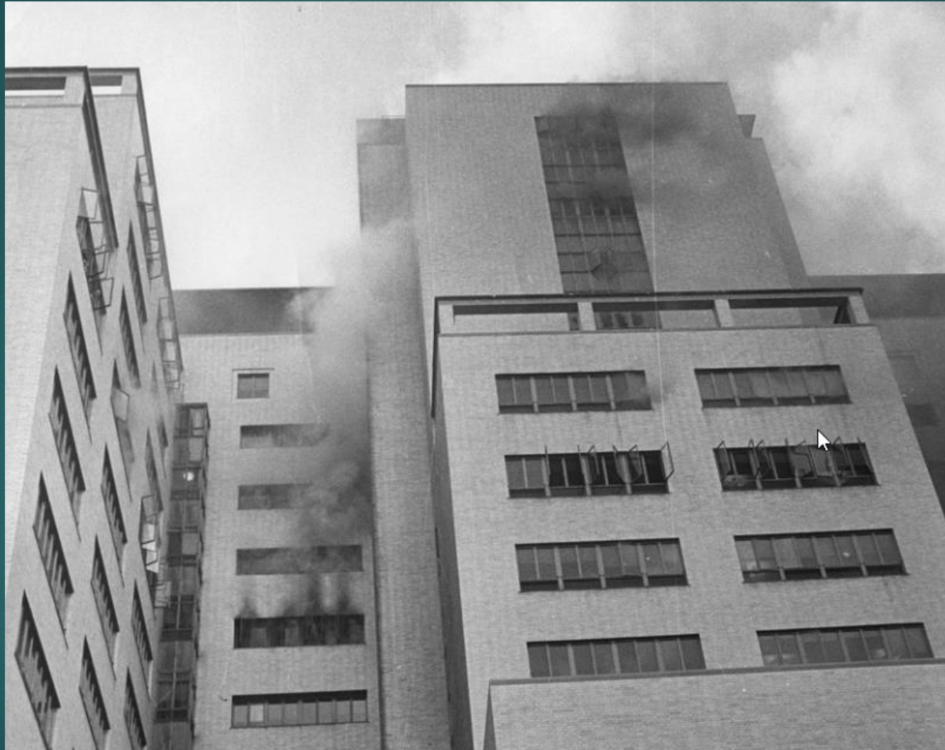
Smoke billows from the ninth floor of Hartford Hospital. Source: The Hamilton Archives at Hartford Hospital.
